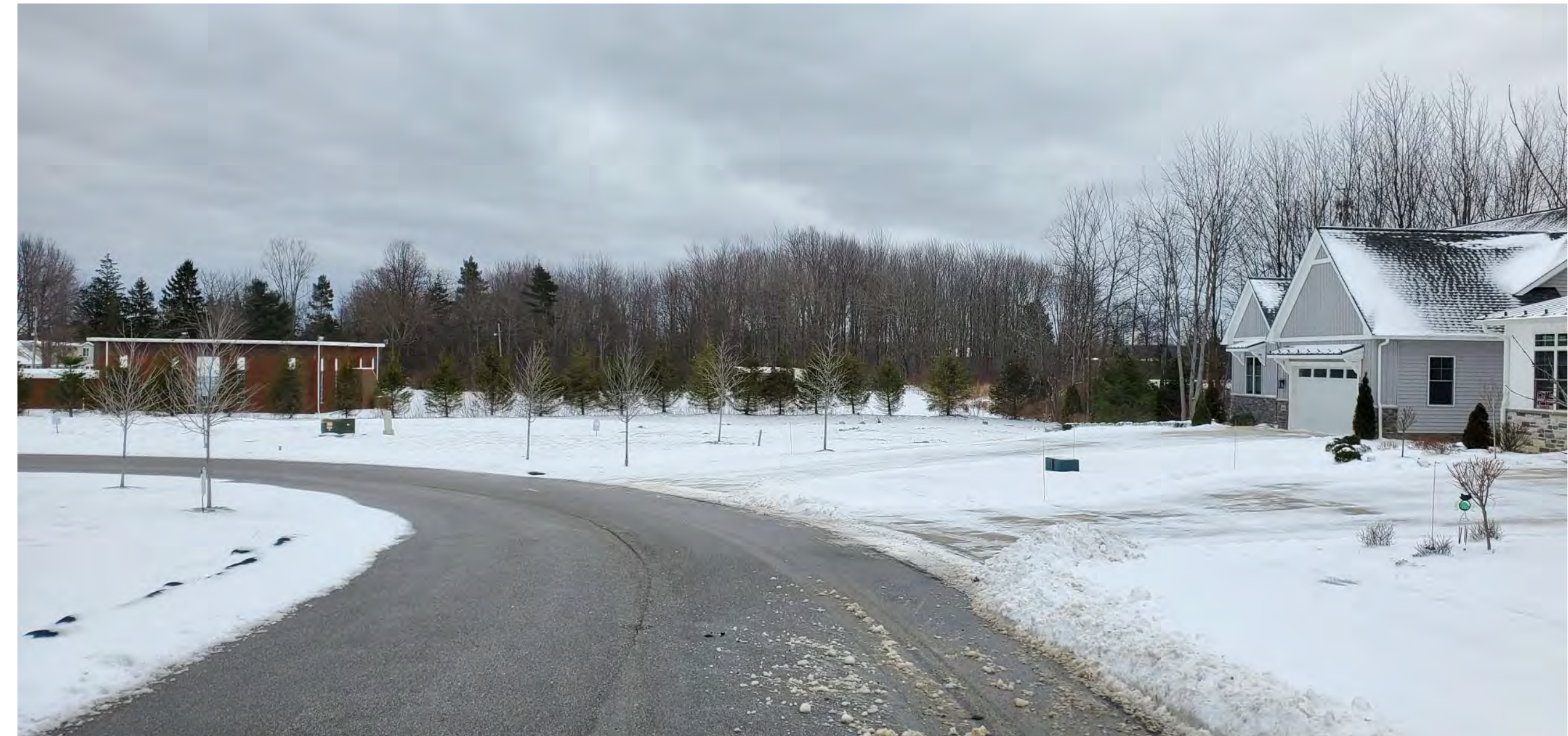
S/L 31 Site From South Cobblestone Rd.
