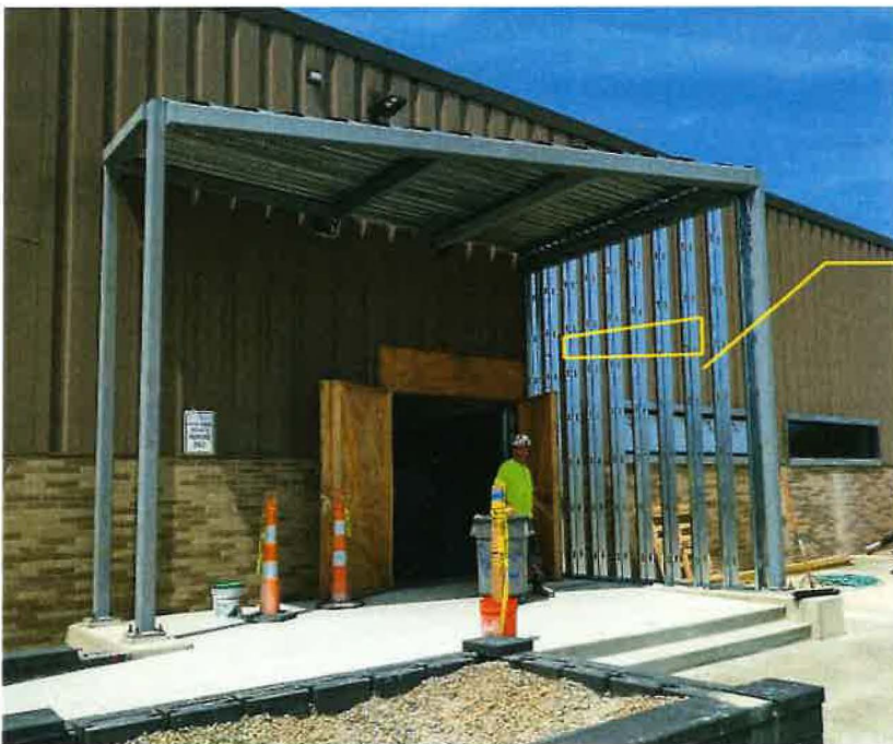
Canopy under construction
