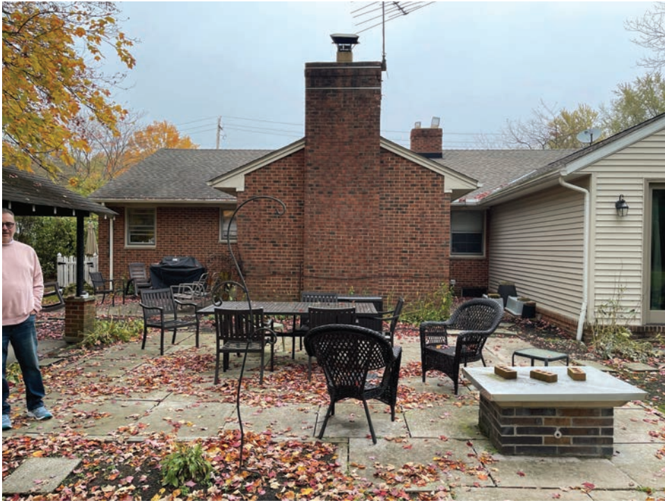
View Looking North at South Elevation
