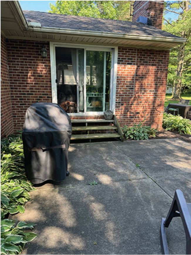
View B- View Looking East at Existing Family Room
